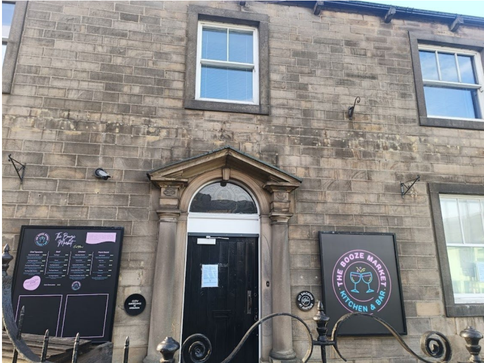
1. The building frontage showing new signage
